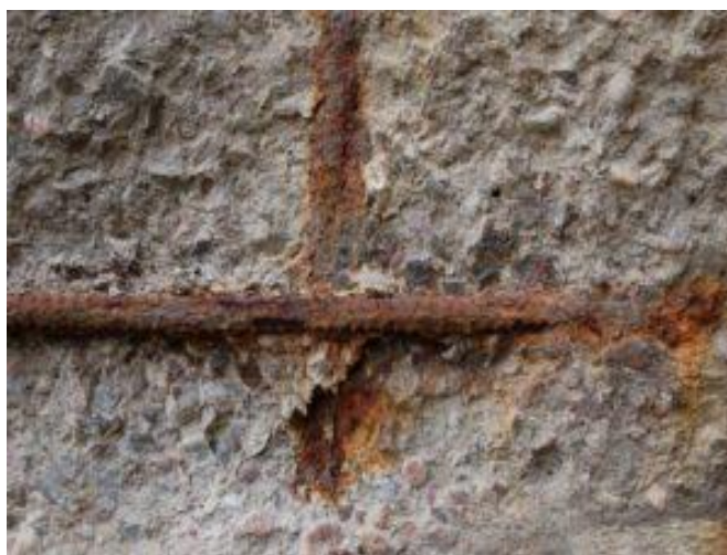
Figure 50. Corrosion
