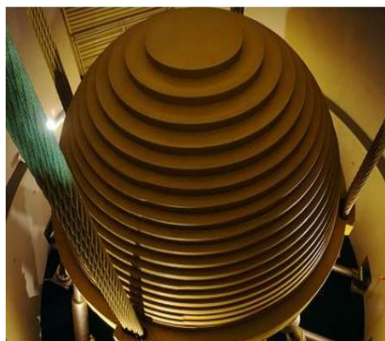
Figure 70 tuned mass damper
